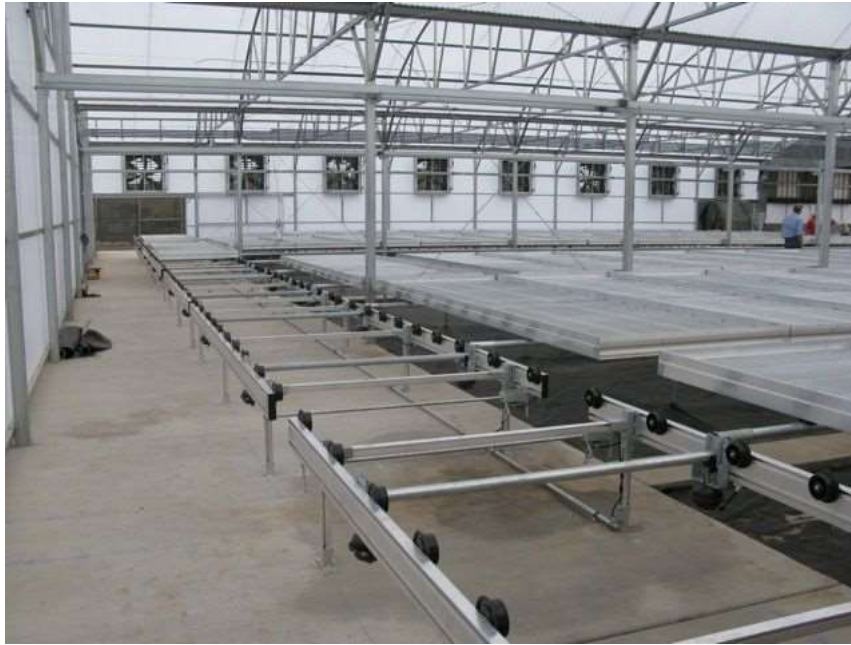
Palletized rolling bench system, which also serves as material handling system
